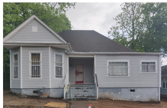
House on Vance in Southside Chattanooga following contamination removal. More than 85 properties have been cleaned up this fiscal year.
